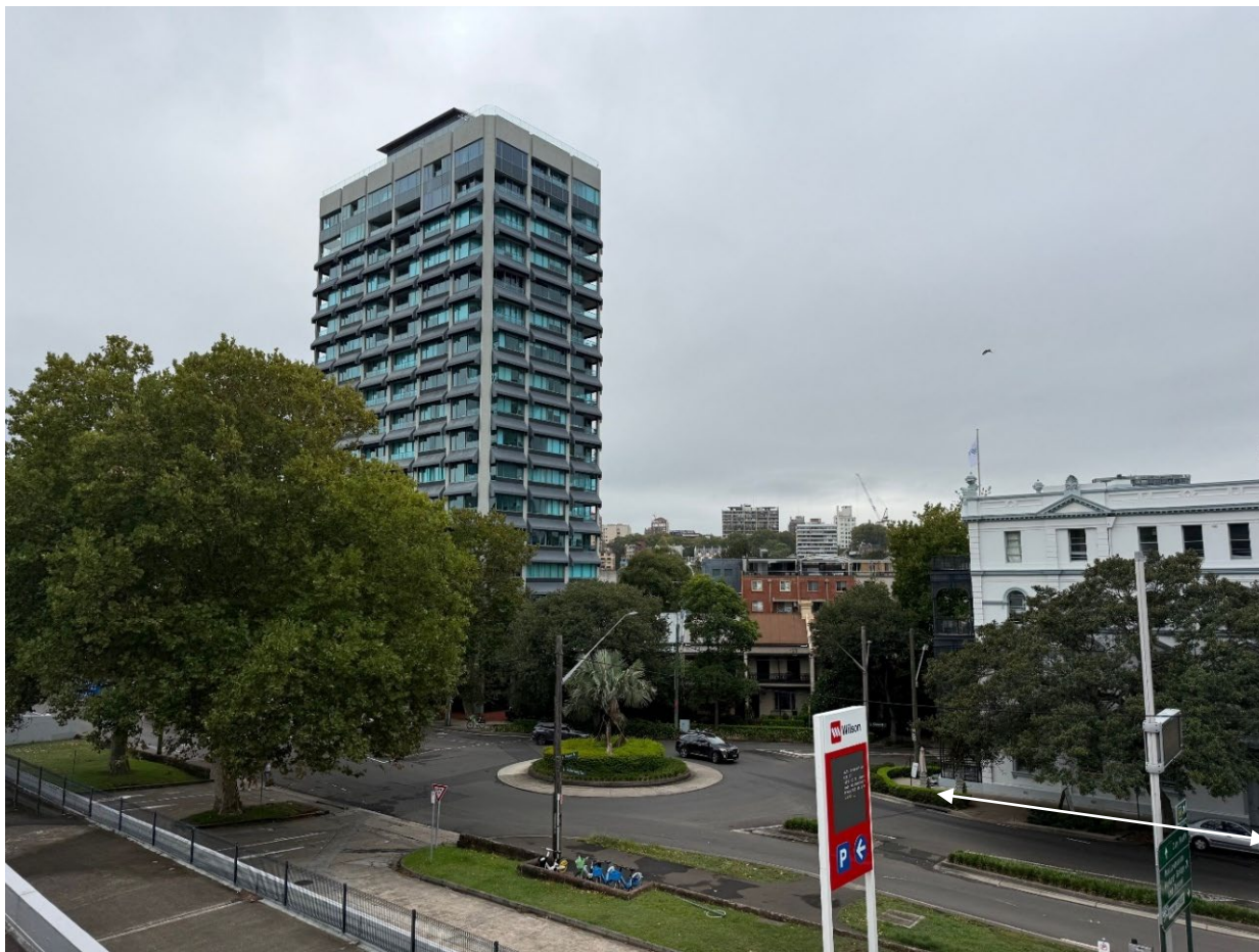
site viewed from the Domain looking north-east
