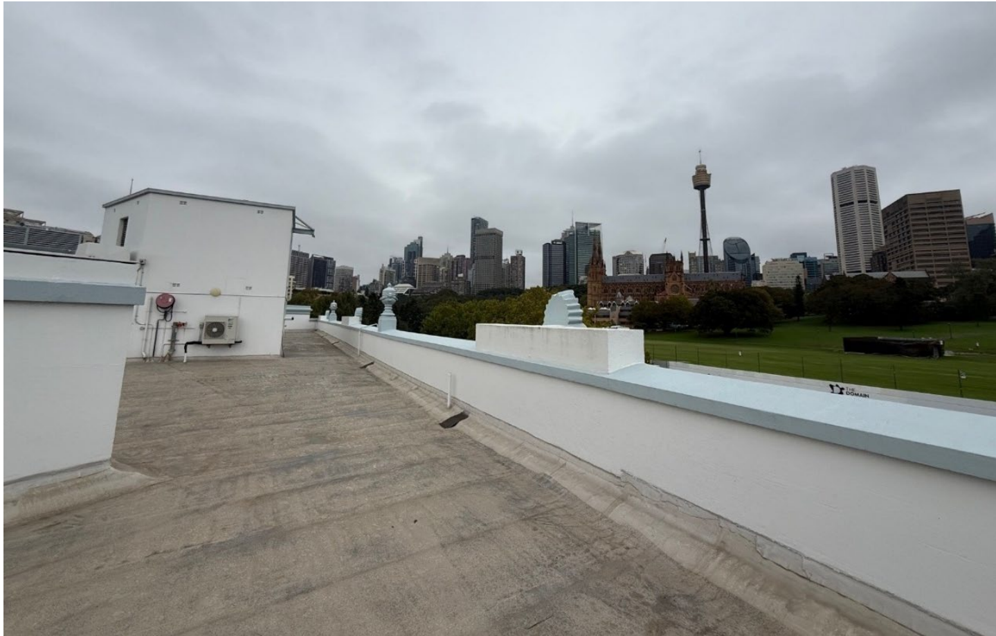
existing rooftop looking south - west
